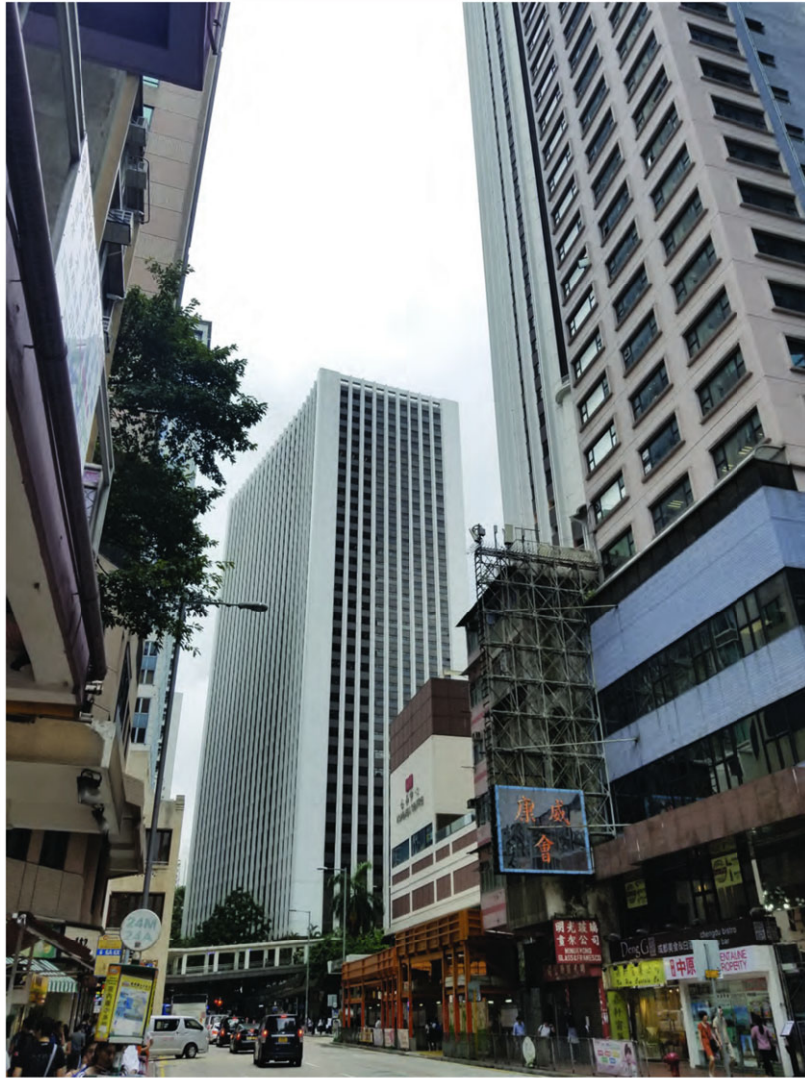
Existing Site Condition at Queen's Road East
