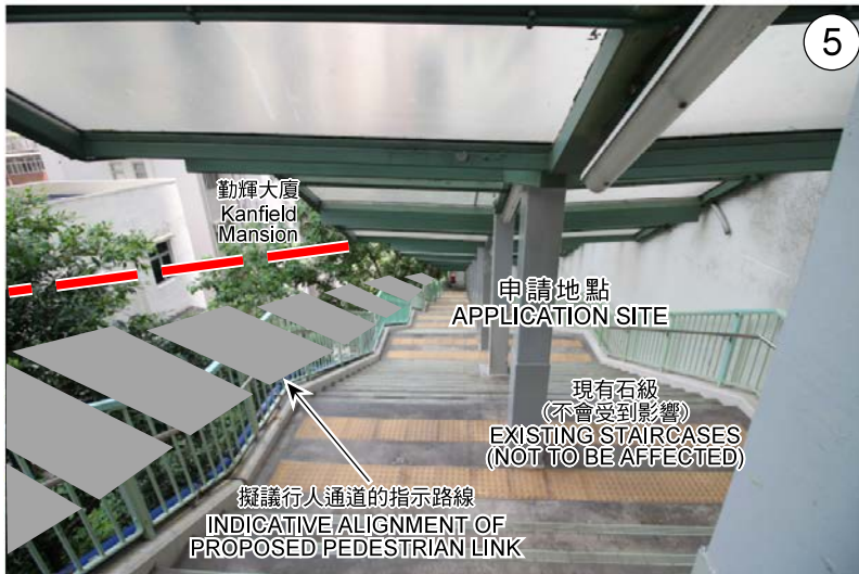
位於浣紗街現有石級通往安庶庇街的申請地點 THE APPLICATION SITE ALONG THE EXISTING STAIRCASES ON WUN SHA STREET TOWARDS ORMSBY STREET
