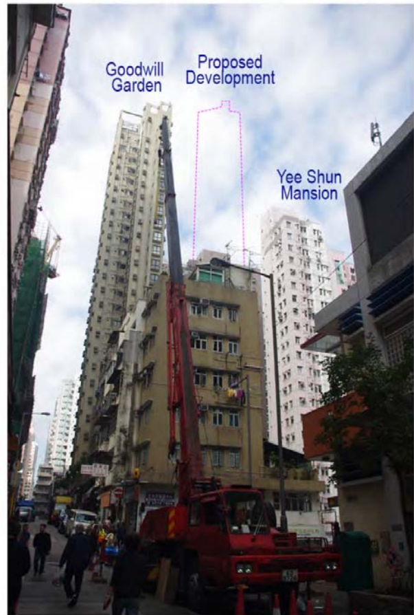
Building Envelope viewed at VP6
