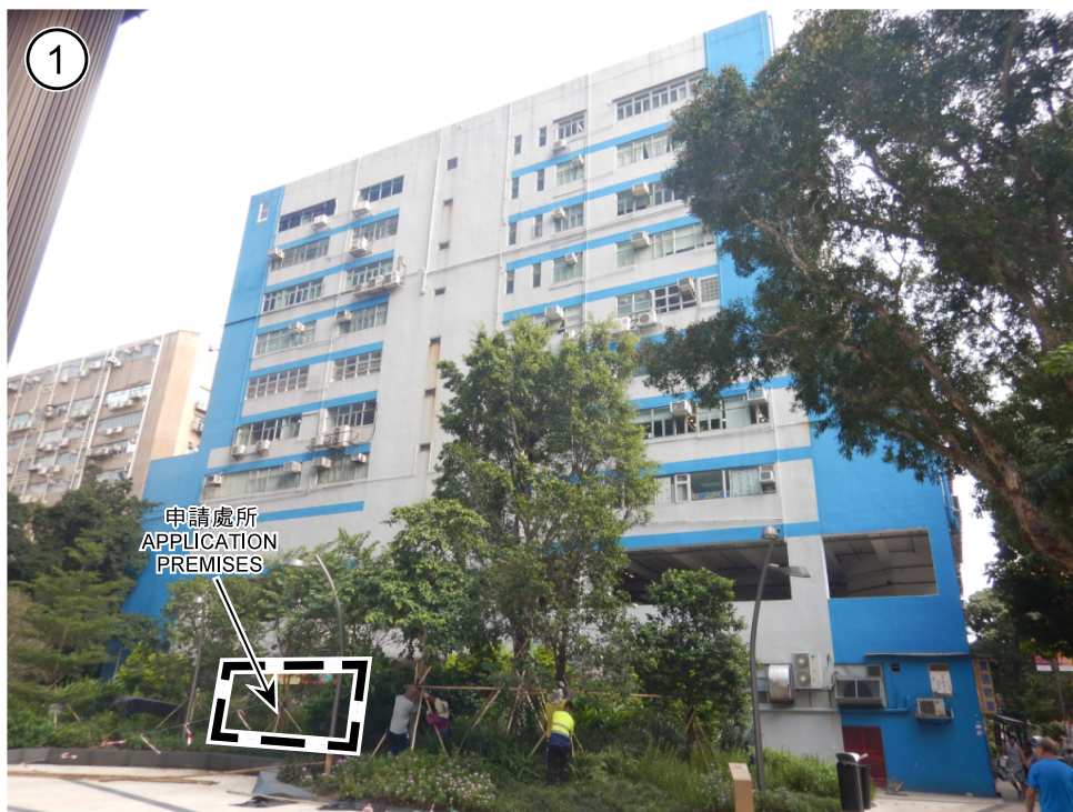
有關樓宇 THE SUBJECT BUILDING
