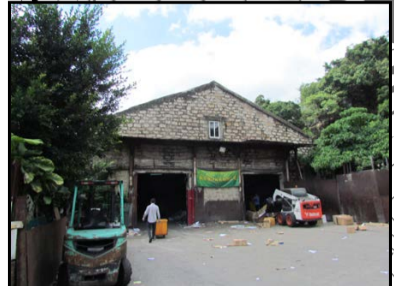
高嶺土採礦廠(1座) Kaolin Mining Plant (Block 1)
