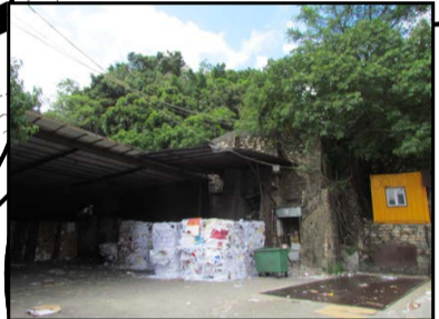
高嶺土採礦廠(2座) Kaolin Mining Plant (Block 2)
