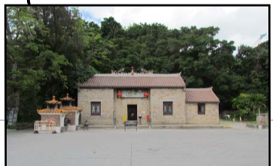
天后古廟 Tin Hau Temple 三級歷史建築 (GRADED 3 HISTORIC BUILDING)
