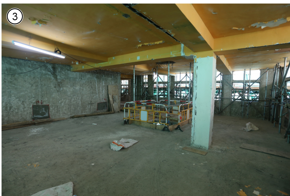
申請處所(十四樓室內) THE APPLICATION PREMISES (INTERIOR AT 14/F)
