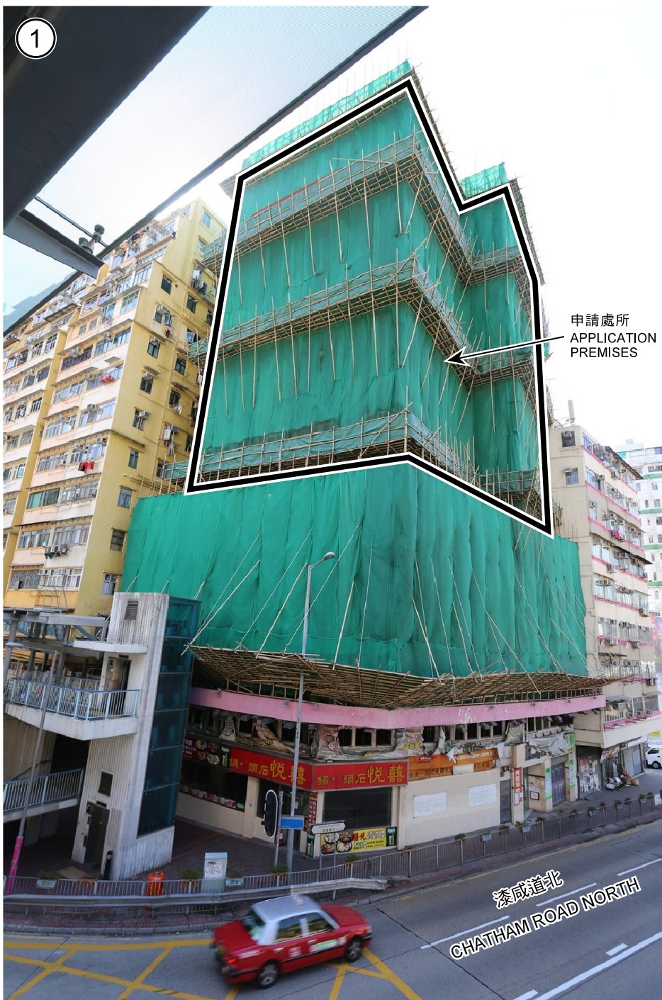
有關樓宇 THE SUBJECT BUILDING
