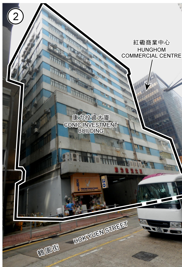
申請地點的現有工業大廈 EXISTING INDUSTRIAL BUILDING AT THE SITE
