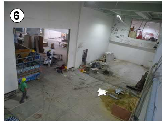
由閣樓拍攝 TAKEN FROM MEZZANINE FLOOR
