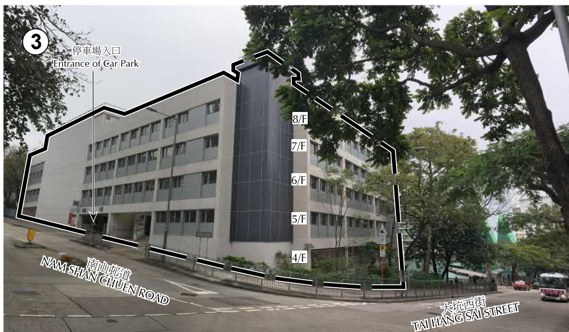
南山邨停車場大樓 CAR PARK BLOCK IN NAM SHAN ESTATE
