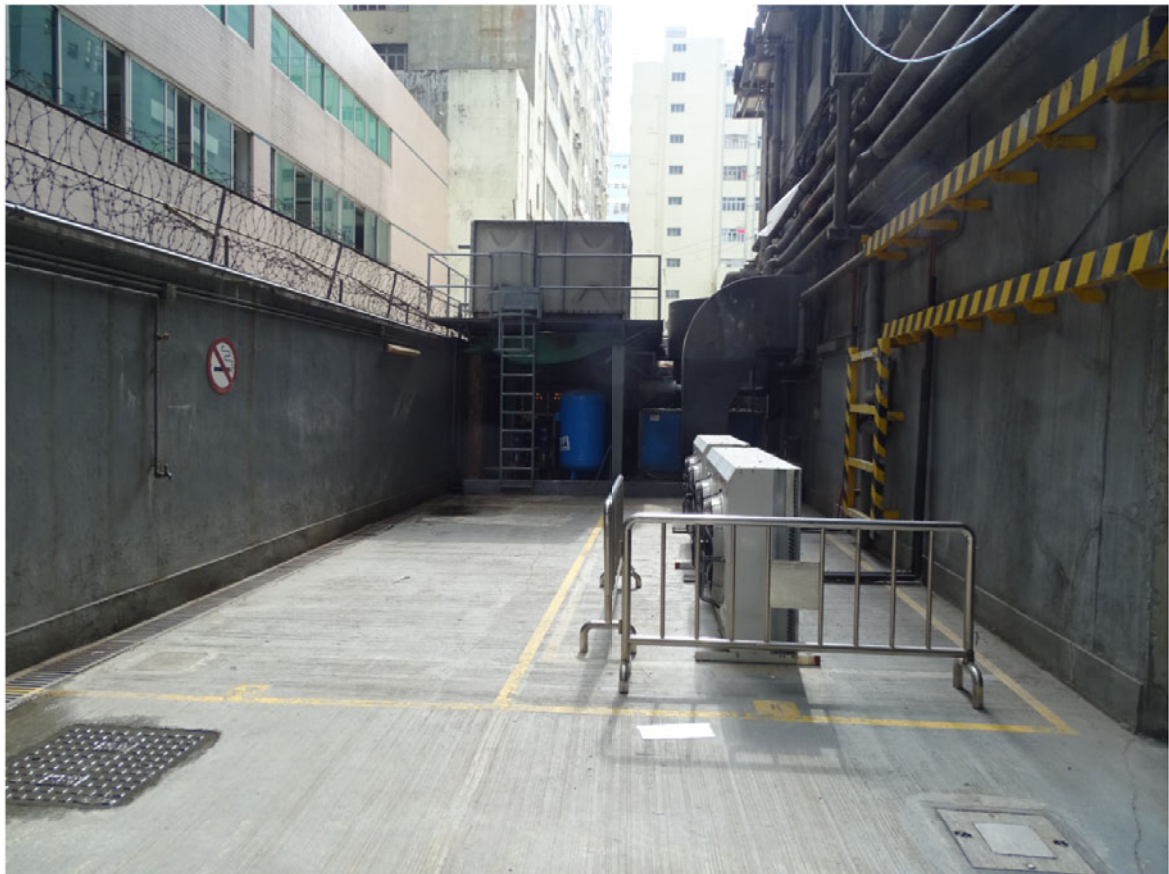
申請處所內部（地下） INTERIOR OF APPLICATION PREMISES (GROUND FLOOR)
