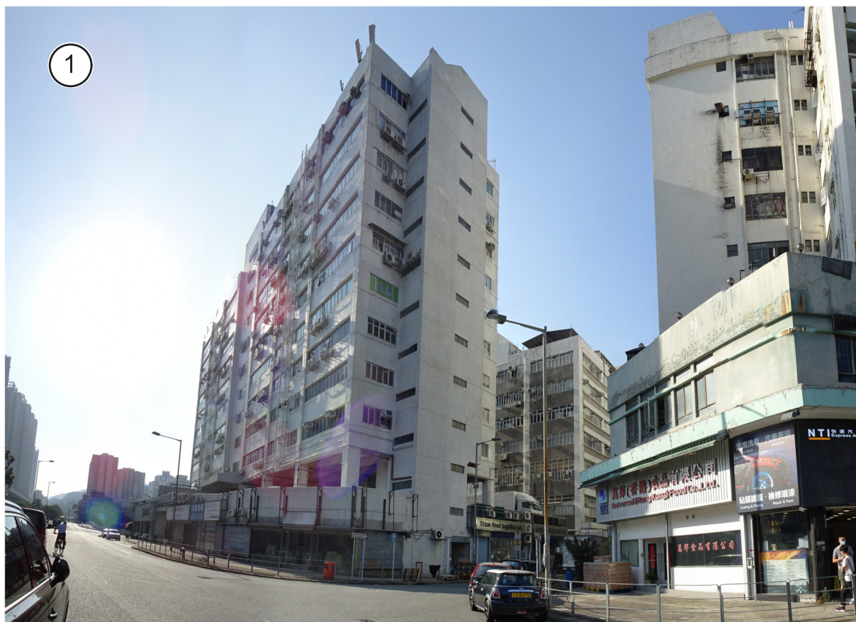
有關樓宇 THE SUBJECT BUILDING
