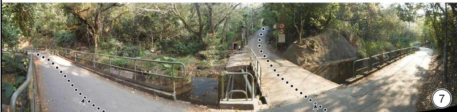
連接荃錦公路的通道 Access Leading from Route Twisk
