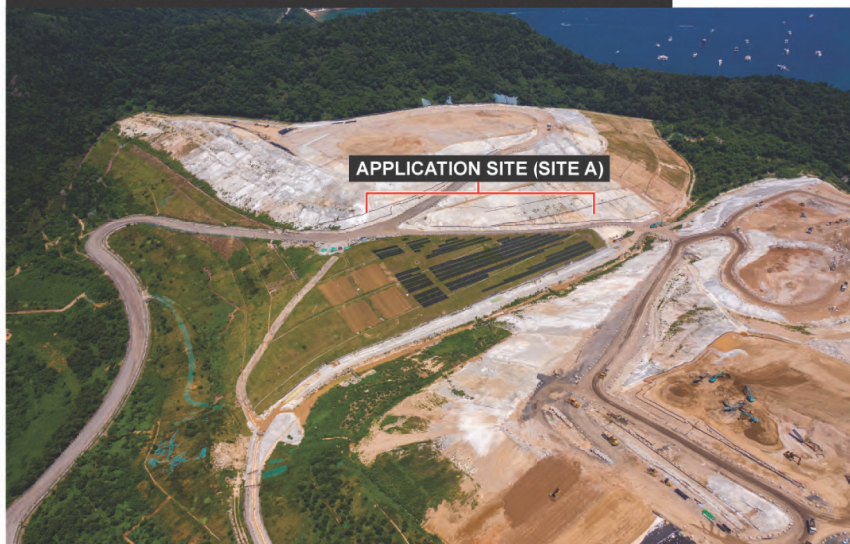
CLOSE UP VIEW ABOVE THE SENT LANDFILL
