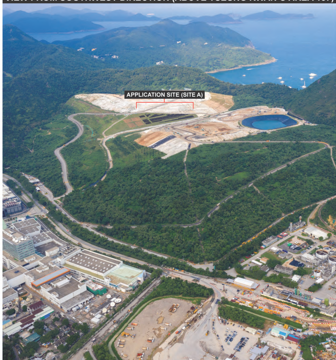
VIEW FROM SOUTHWEST DIRECTION (ABOVE TSEUNG KWAN O AREA 137)
