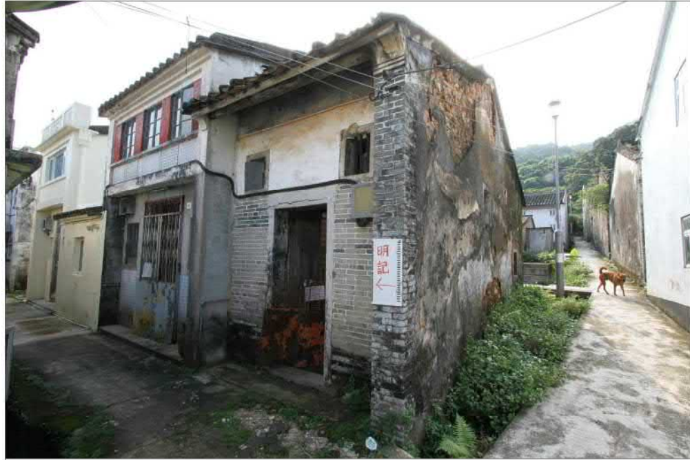
HOUSE LOT 200 BEFORE RESTORATION
