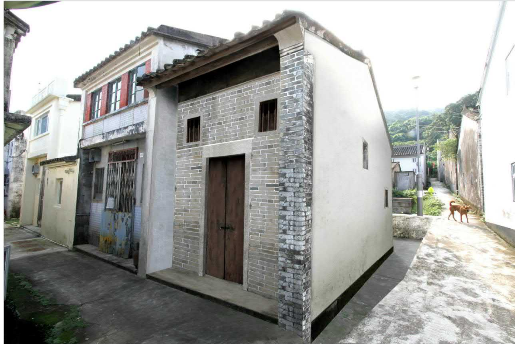
HOUSE LOT 200 AFTER RESTORATION
