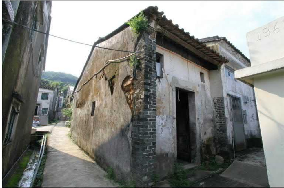
HOUSE LOT 286 S.A. BEFORE RESTORATION
