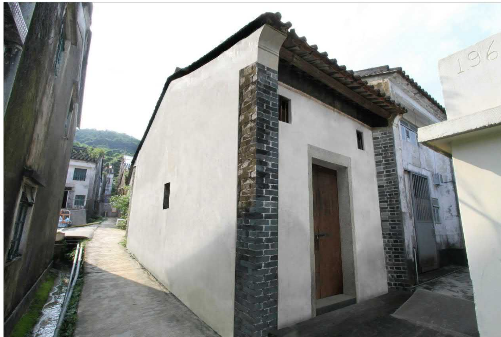
HOUSE LOT 286 S.A. AFTER RESTORATION
