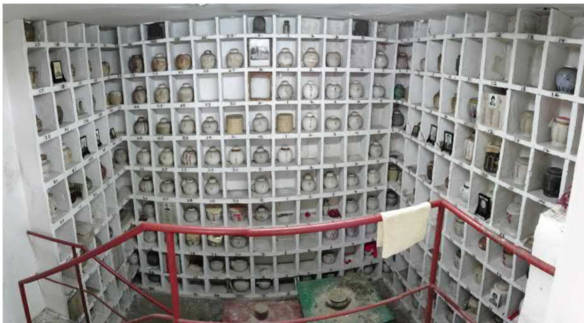
構築物編號 16 (壁龕) (設有靈灰龕位) Structure No.16 (with Columbarium Niches)
