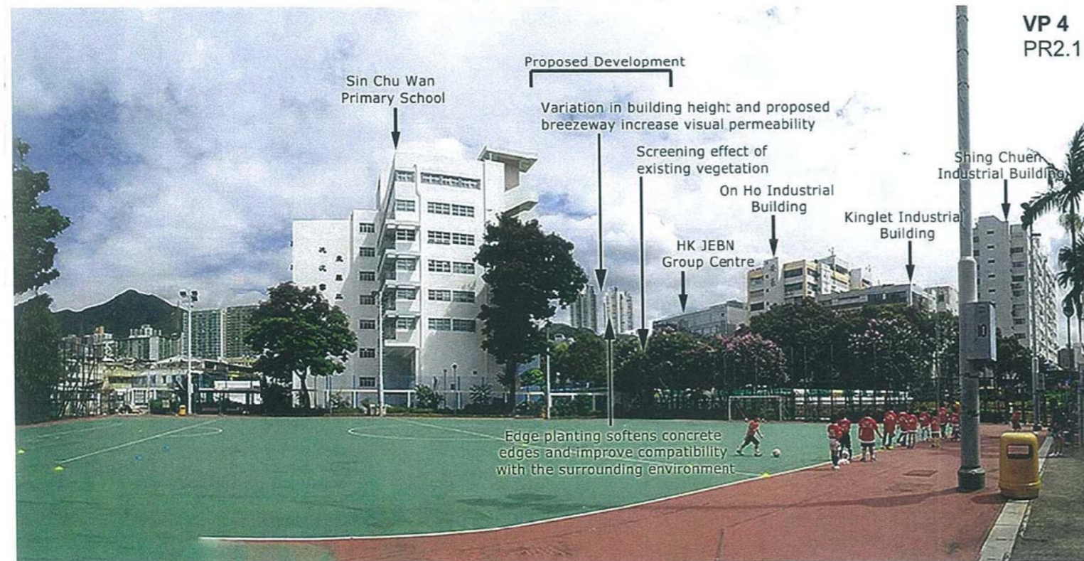
VP4 : VIEW FROM CHIK LUK LANE BALLCOURT (Year 10 of Operational Phase)
