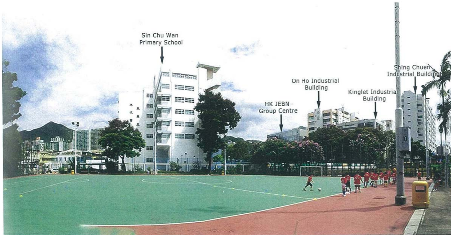
VP4 : VIEW FROM CHIK LUK LANE BALLCOURT (Existing Condition)
