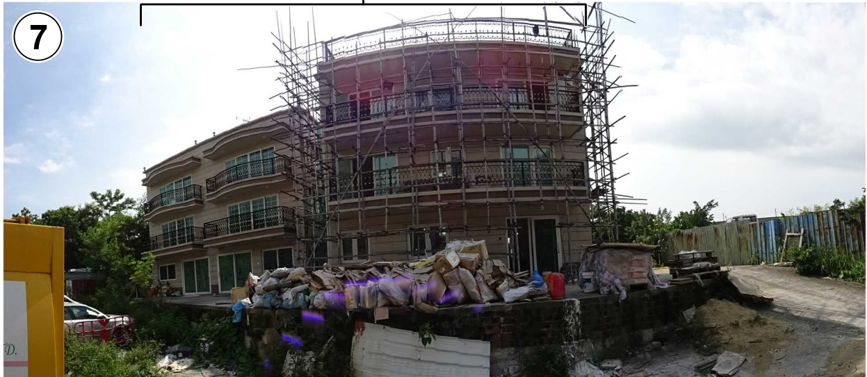
住用屋宇(裝修中) Residential House (Under Renovation)
