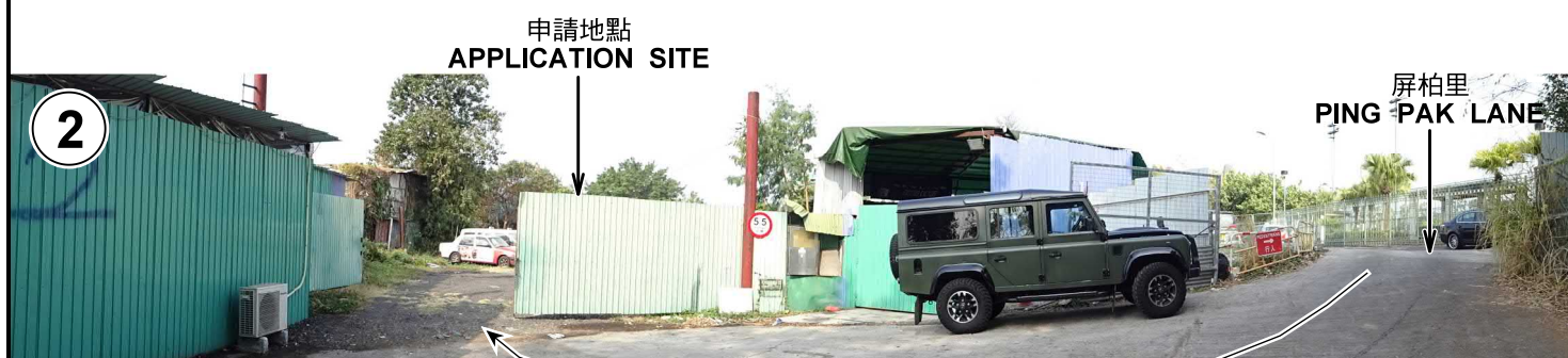
連接屏柏里的通道 Access Leading from Ping Pak Lane
