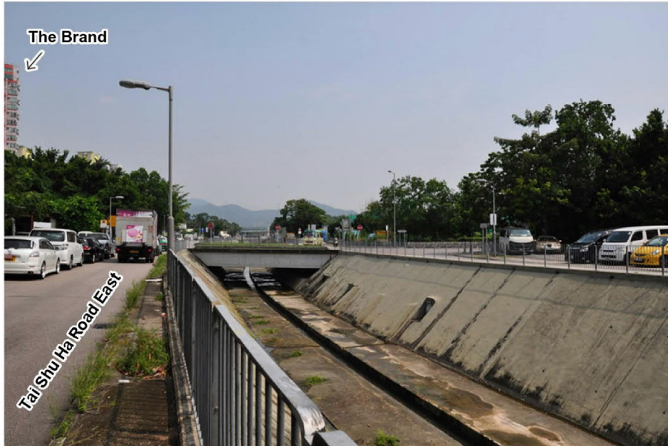
Photo 3 Existing Condition at the Application Site
