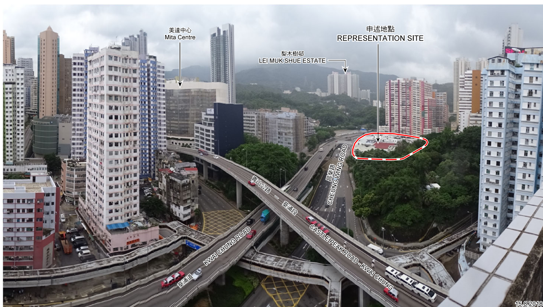
由南面觀望的景觀 VIEW FROM THE SOUTH
