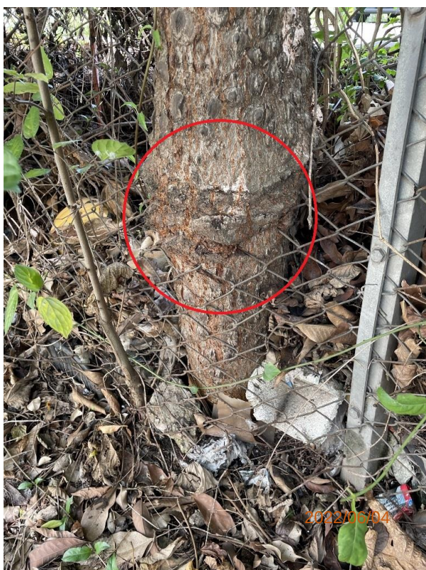
T23 Wire Enveloped in Trunk - FELL
