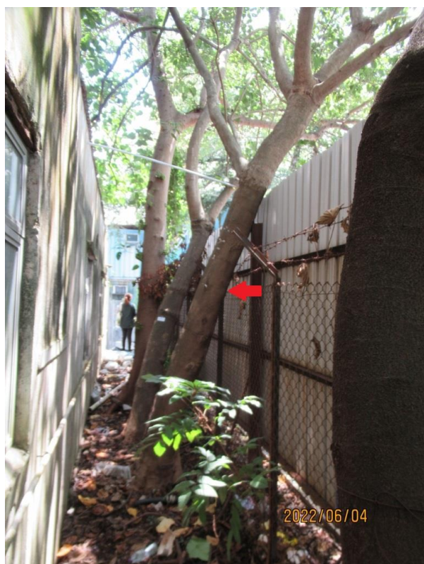
T6 Trunk Condition - FELL
