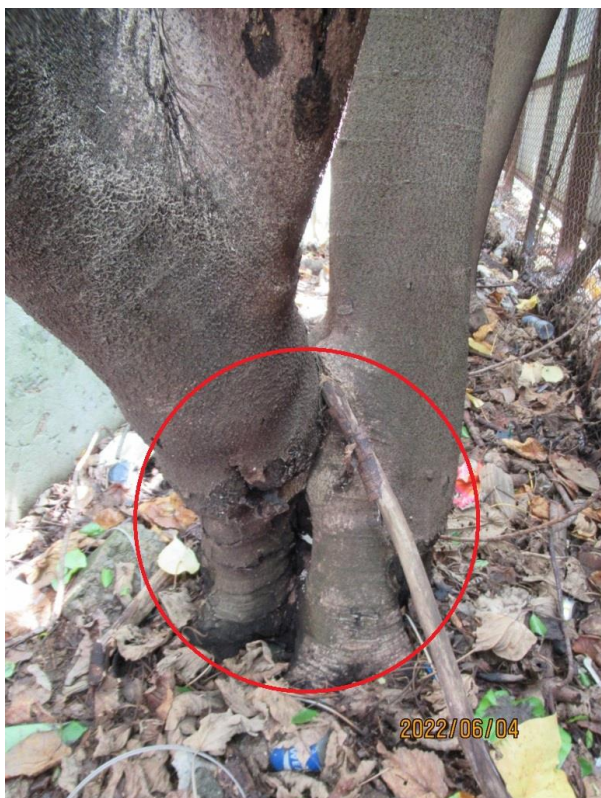
T9 Codominant Trunks with Included Bark Decay - FELL
