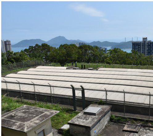
VP09: LR9 Infrastructural Development
