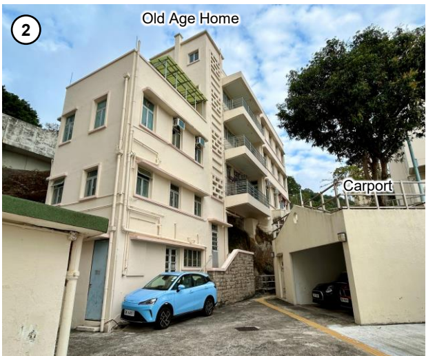
View Towards the Old Age Home and Single-Storey Carport
