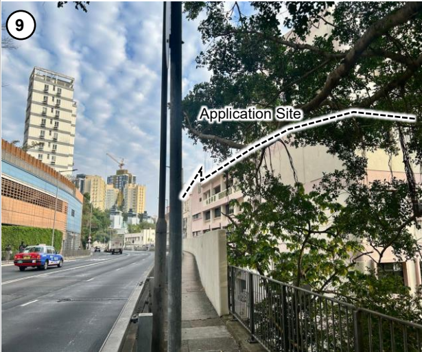
View of the Application Site from North-West Direction from Pok Fu Lam Road
