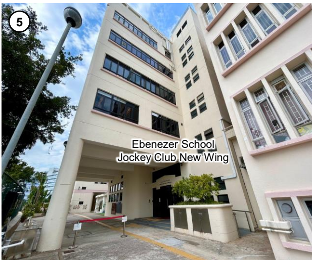
View Towards the New Ebenezer School Jockey Club New Wing
