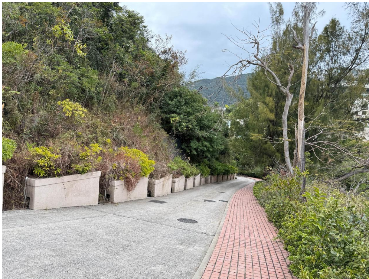
Photo 3: General view of the access road
