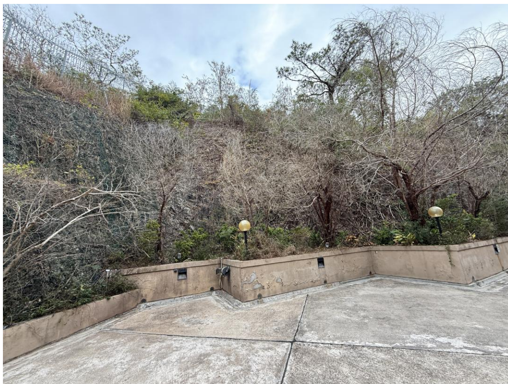
Photo 2: General view of Feature 11SW-D/C1854
