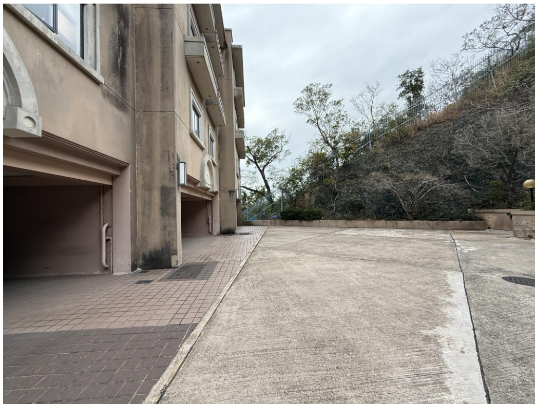
Photo 1: General View of site
