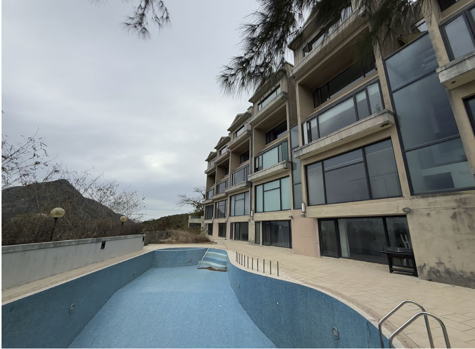
Photo 3 – Existing Swimming Pool Environment
