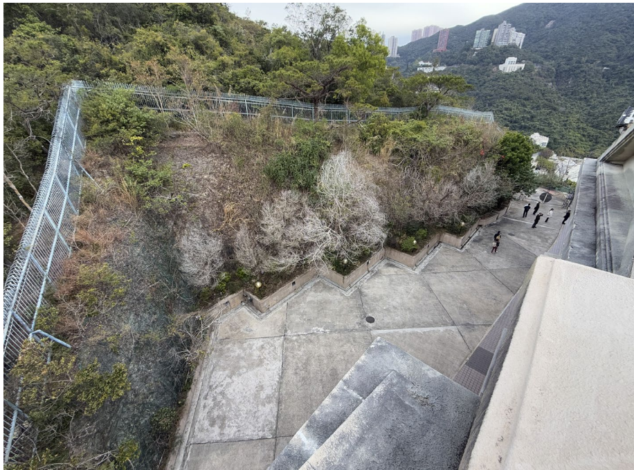
Photo 2 – Photo of Driveway and Main gate taken from rooftop of existing units
