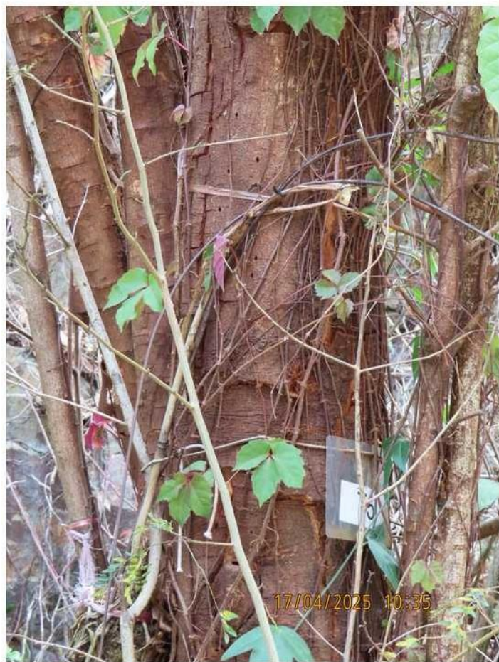
T5_Dead tree (Loose bark) (3)
