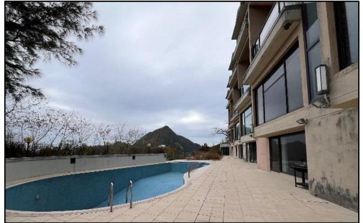
Photo 2.2 Existing Site Condition as viewed from the Lower Platform
