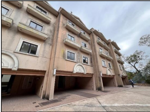
Photo 2.1 Existing Site Condition as viewed from the Main Entrance
