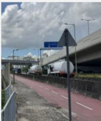
Narrow footpath along Kiu Cheong Road with no shading and trees
