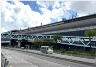
Long ramp outside Exit B of TSW Station
