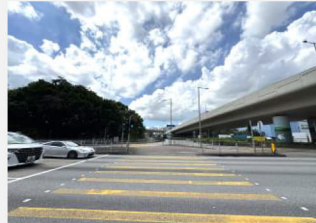
Signal-controlled crossings at J/O Hung Tin Road & Ping Ha Road
