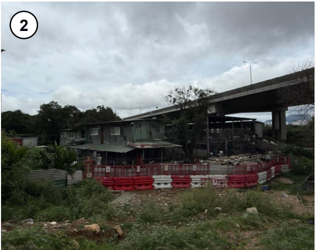
Existing Temporary Structures
