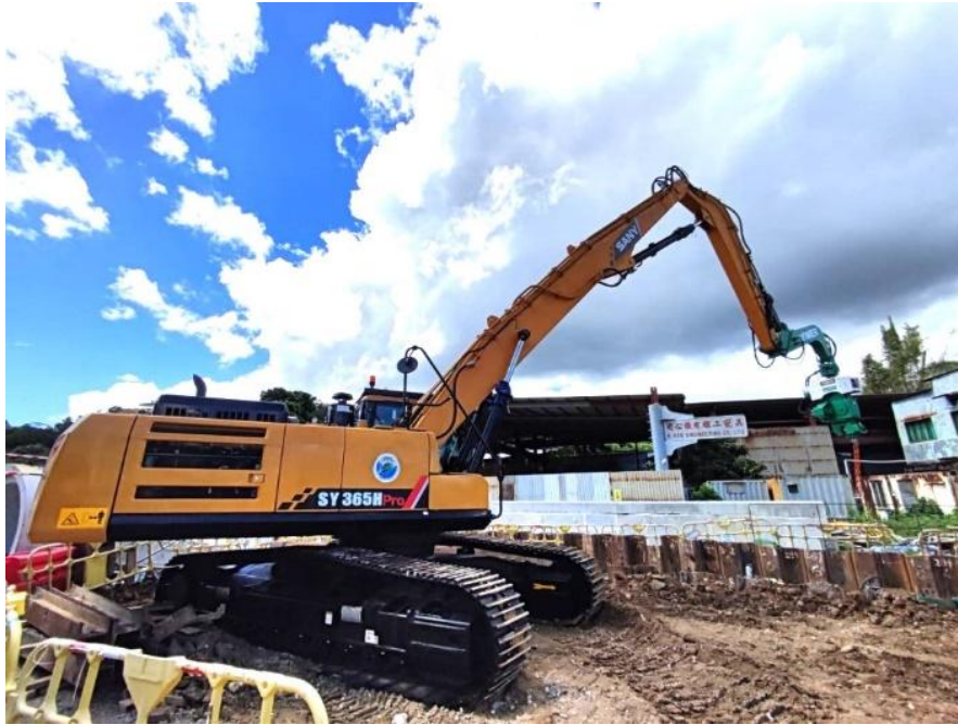
Photo 1: Heavy specialized machinery for installation of sheet pile
