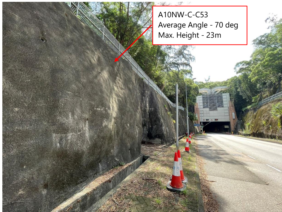
Photo 2: General View of 10NW-C-C53
