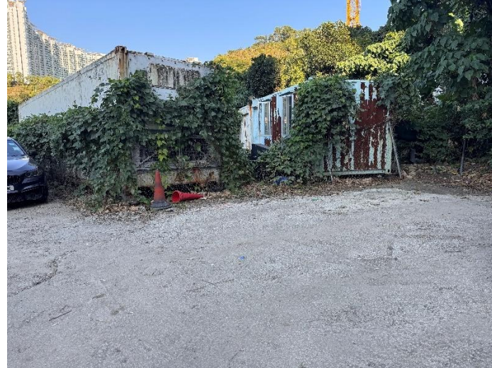
Photo 2: Storage containers are observed. However, there are no direct contact between the containers and the ground and the ground is paved with concrete in good condition. No oil stains and smells are observed.
