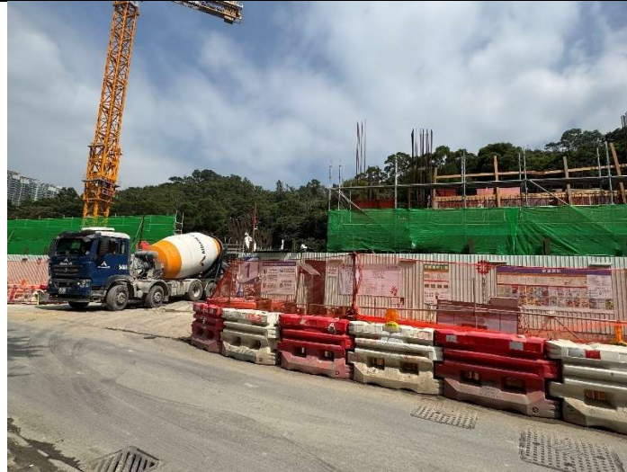
Public Housing Development at Tung Chung Area 23, Housing Department
