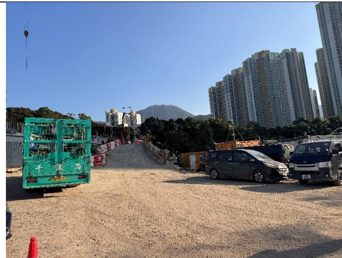
Photo 8: Entrance road of the Site. The area is covered with sand in good condition. No oil stains and smells are observed.
