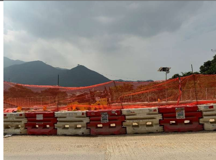
Road Improvement Work at Tung Chung Road North
