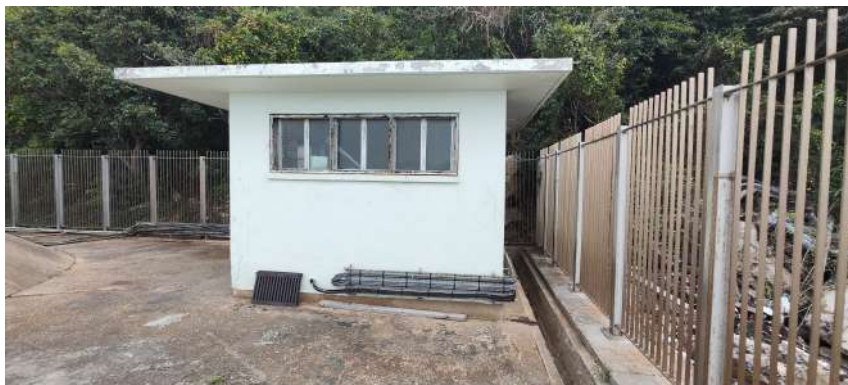
Figure 14: DSD technical room.
