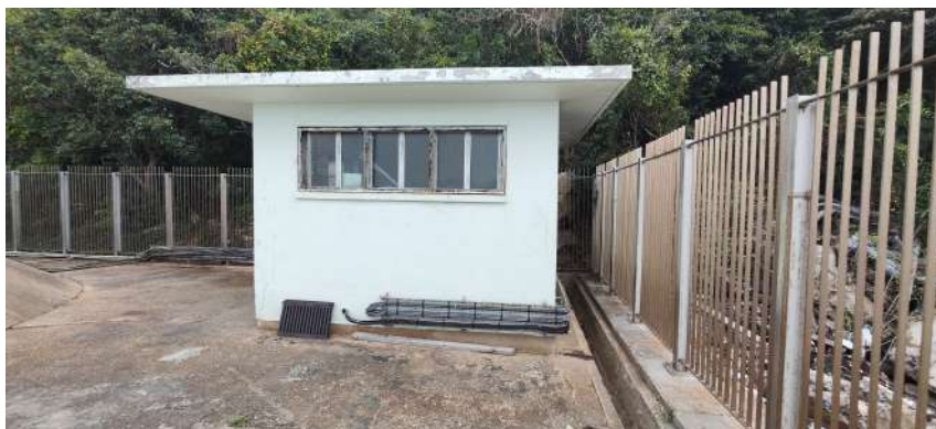
Figure 14: DSD technical room.
