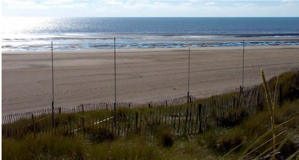
Figure 7 Antenna Array along a public beach in Liverpool Bay, UK
