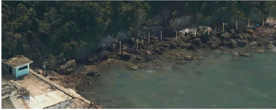
Figure 9 Rendering showing the antennas on Tai O Wastewater Treatment
