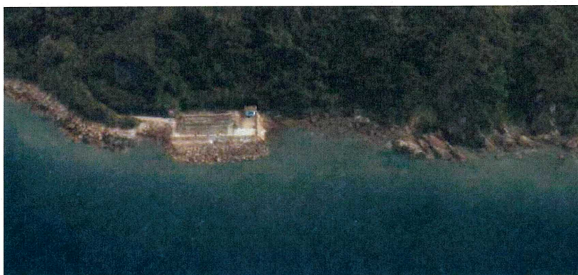
Figure 9: Aerial view of Tai O - Wastewater Treatment Station site.
