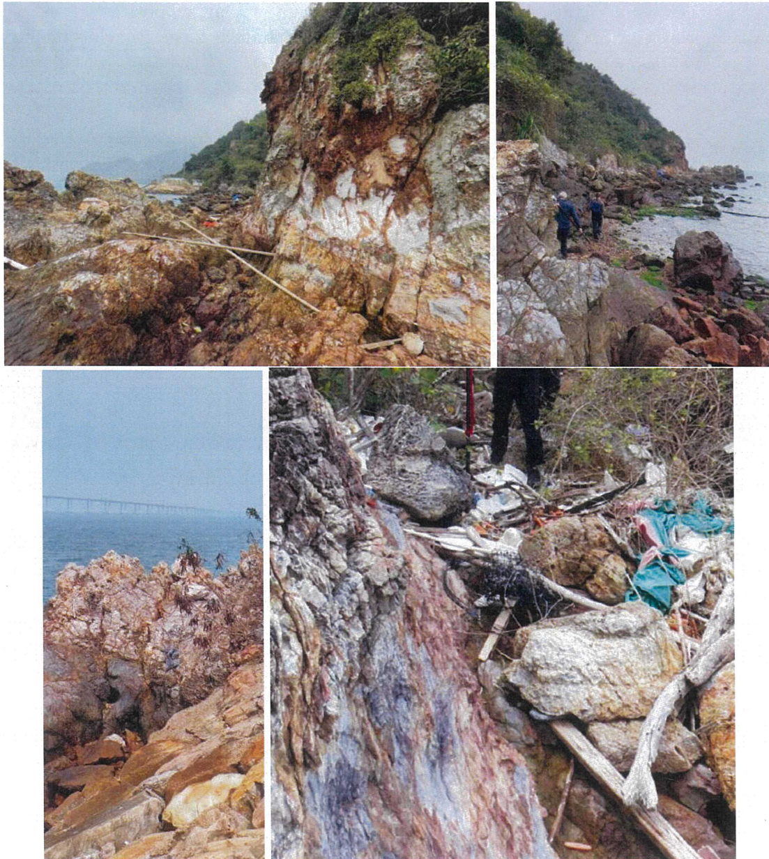
Figure 12: Station Tai O Wastewater Treatment Current State. Top left: view from the last Rx toward the Wastewater Plant Station; Top right: view toward the Rx position from the Wastewater Plant Station; Bottom left: Tx positions (Wastewater Plant Station on the back); Bottom right: accumulation of garbage due to flooding.
