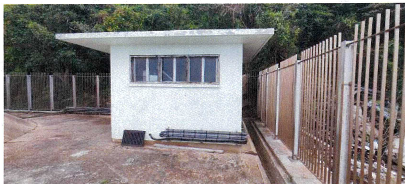
Figure 14: DSD technical room.
