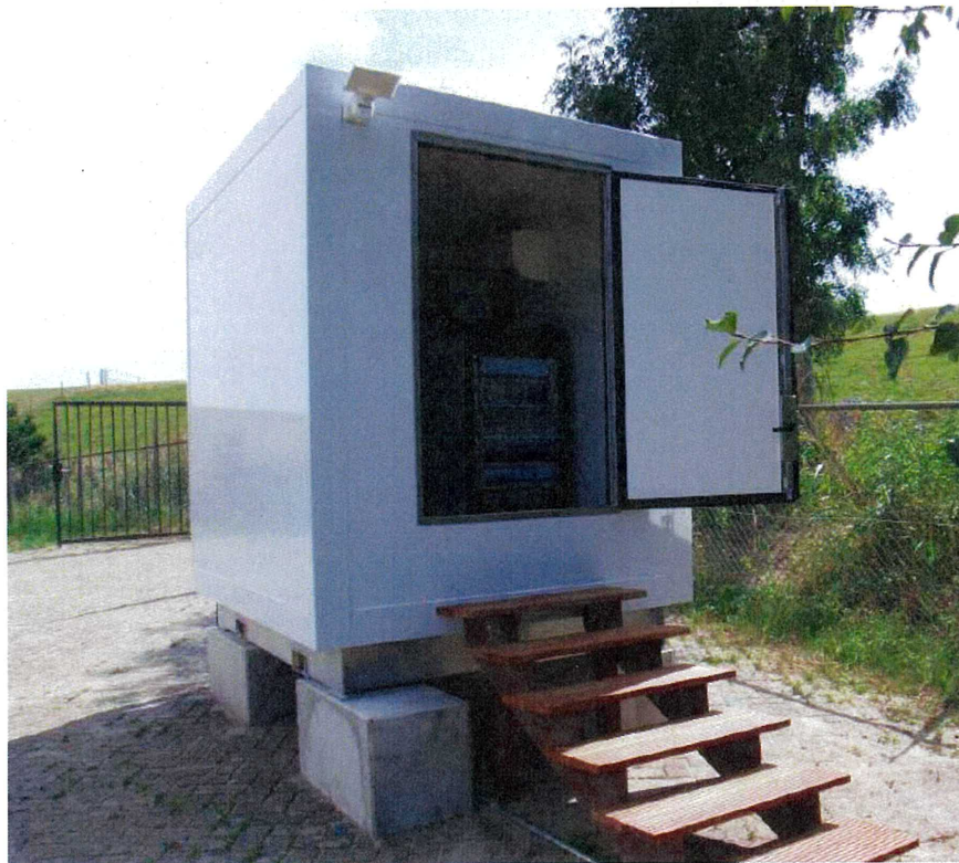
Figure 7: Example of a small portable cabin, used as local server room.
