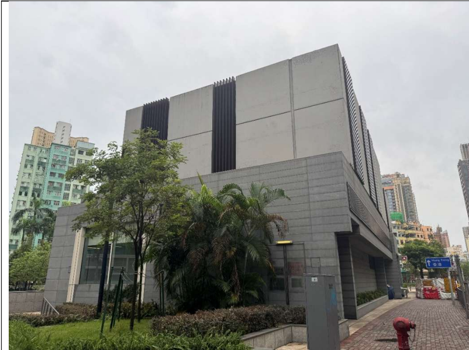
E01 to E17 To Kwa Wan MTR Station Exit D – Ventilation Louvre and Cooling Tower Operation follow MTR operation hour (Both daytime & evening time and night-time operation) SWL reference from FPNAR of To Kwa Wan Station under SCL
