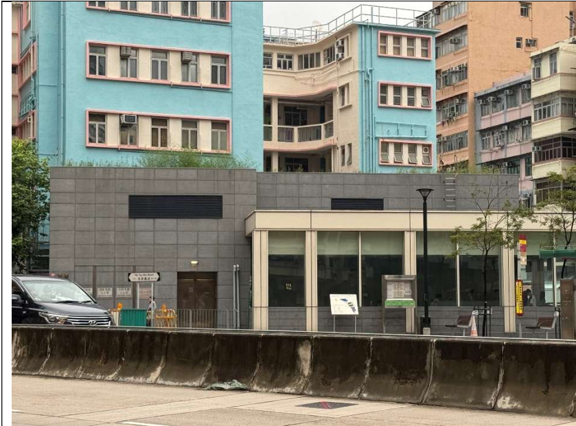
H01 to H06 To Kwa Wan MTR Station Exit A (next to To Kwa Wan Market) – Ventilation Louvre Operation follow MTR operation hour (Both daytime & evening time and night-time operation) SWL reference from FPNAR of To Kwa Wan Station under SCL
