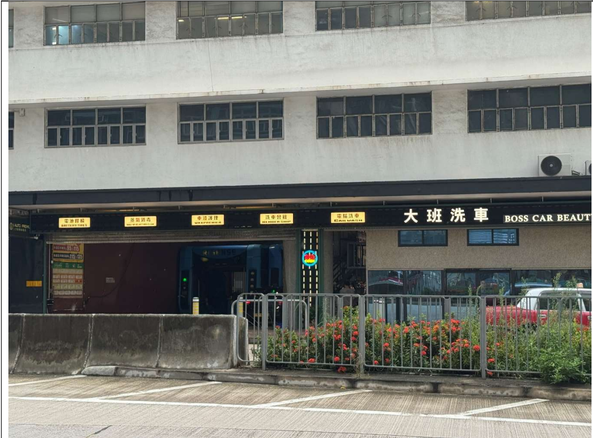
G01 Gainfall Centre – Car Washing 24-hour operation SWL reference from EA report of HSK/HT NDA
