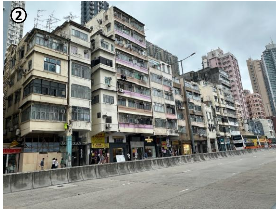
Views of the Application Site from Ma Tau Wai Road
