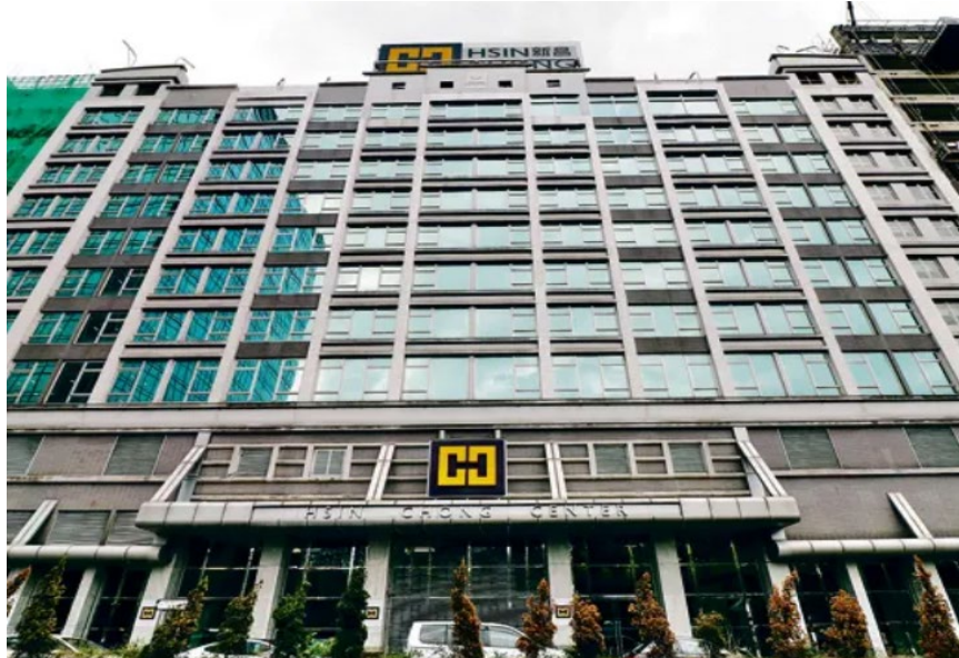
Hsin Chong Centre (office building) taken in 2017
