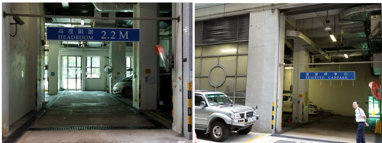
Internal transport facilities on G/F of Hsin Chong Centre taken in 2017
