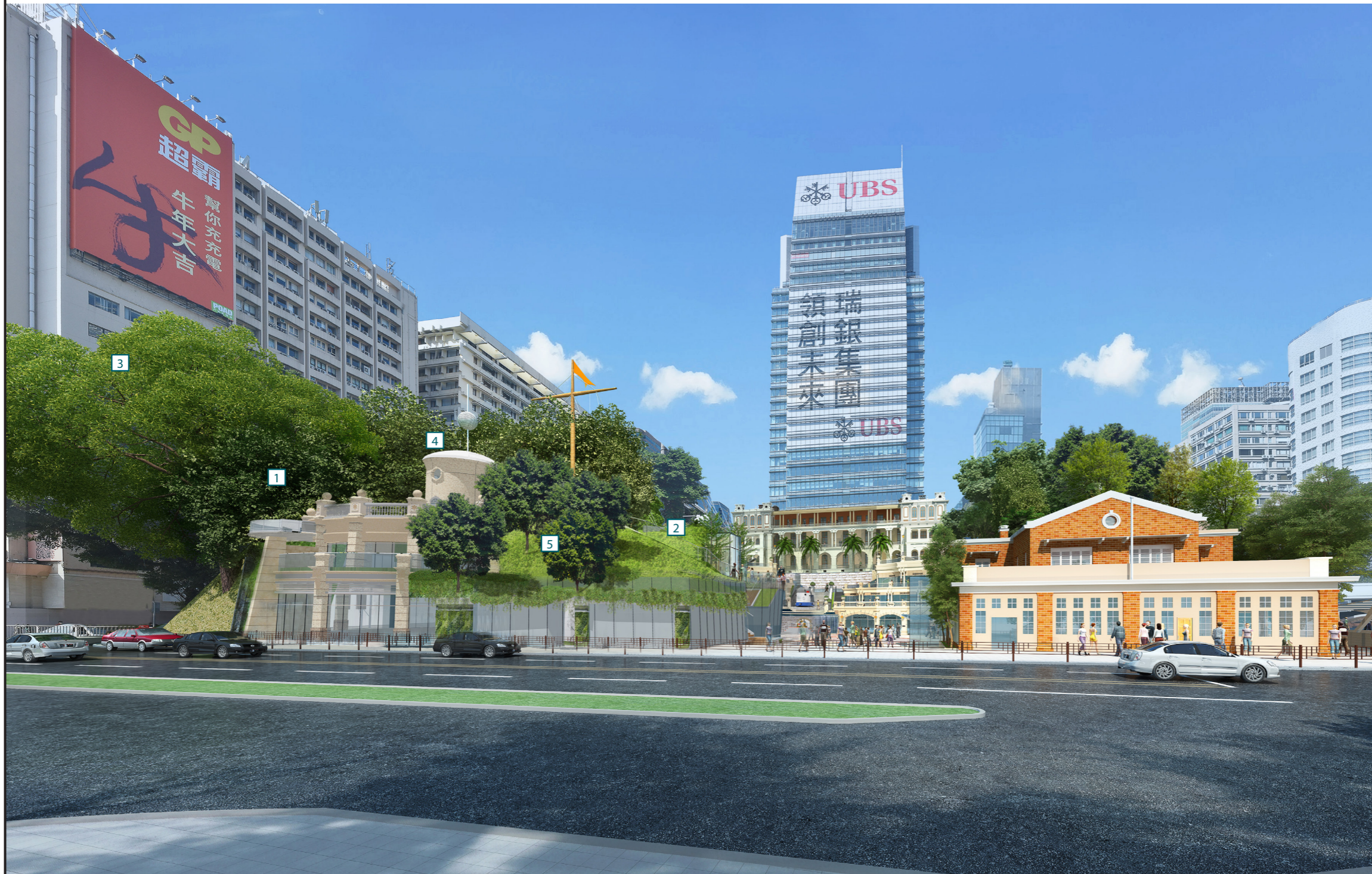
Pedestrian level view from Salisbury Road to the south
