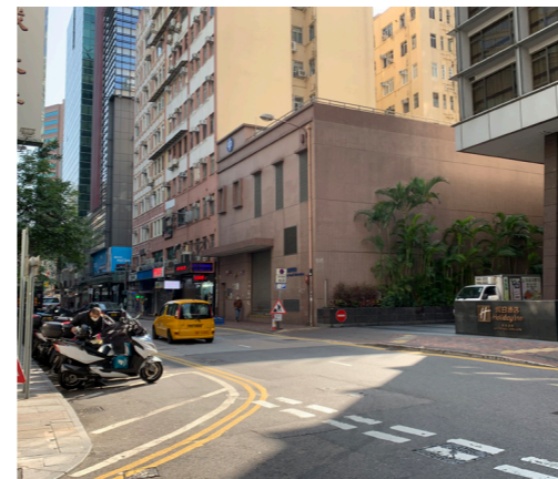
VP11: LR10 Infrastructure
