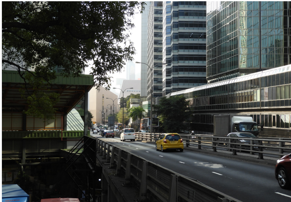
A Views from the north towards the site area are largely obscured by commercial developments alongside Kowloon Park Drive.
