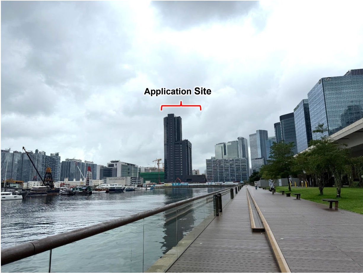
Figure 2.2a Site Photo (Viewing from Kwun Tong Promenade)
