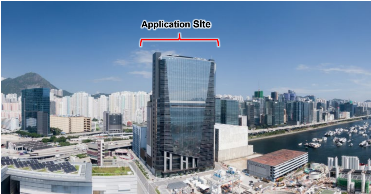
Figure 2.2b Site Photo (Viewing from southwest)
