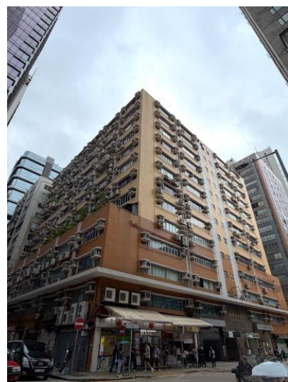
6 Wing Kut Industrial Building
