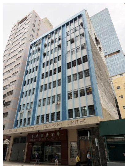
3 Yick Tai Industrial Building
