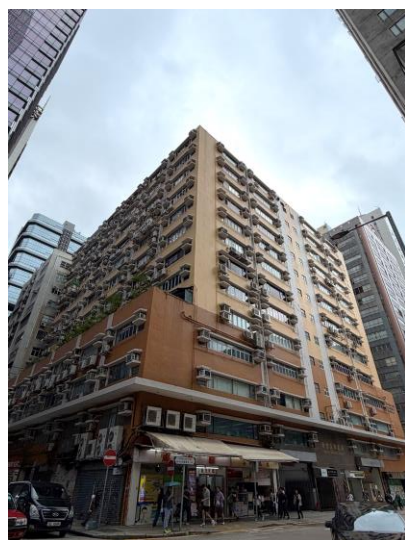
6 Wing Kut Industrial Building
