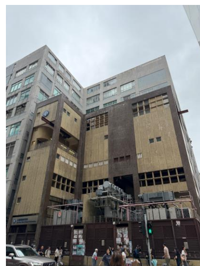
5 Tai Nan West Street Substation
