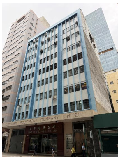
3 Yick Tai Industrial Building
