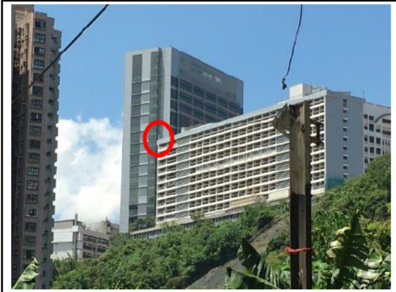
Photo 7.3: Chimney at rooftop of Kwai Chung Hospital
