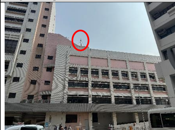
Photo 7.2: Chimney at rooftop of Princess Margaret Hospital
