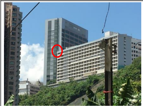
Photo 7.3: Chimney at rooftop of Kwai Chung Hospital
