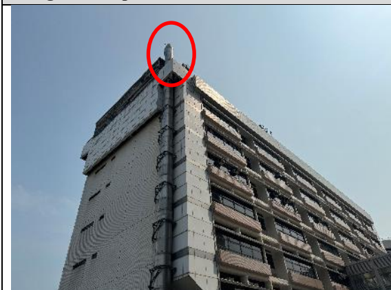
Photo 7.1: Chimney at rooftop of Princess Margaret Hospital
