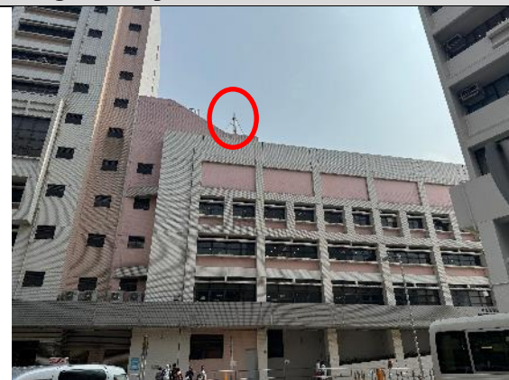
Photo 7.2: Chimney at rooftop of Princess Margaret Hospital
