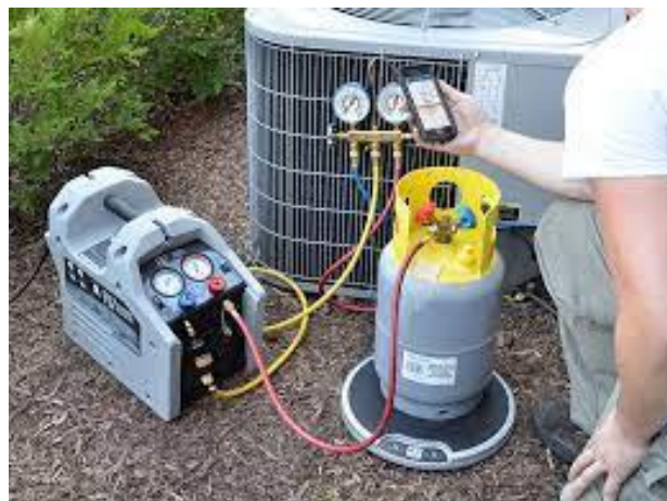
Figure 3. Application of refrigerant recycle system on chillers
