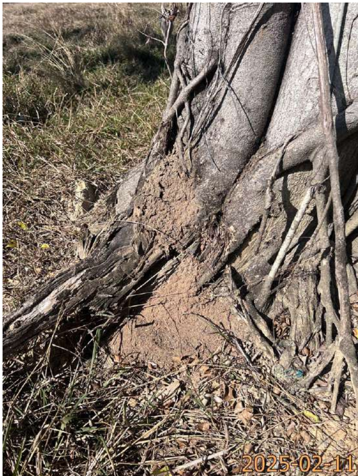
T17 Trace of termite
